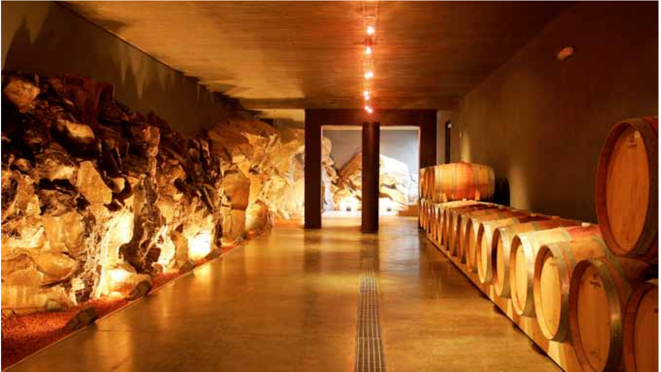
Still more than enough rock in the barrel cellar: the dramatic, jagged wall of blue-gray granite left after the detonation of more than 220lb (100kg) of explosives
